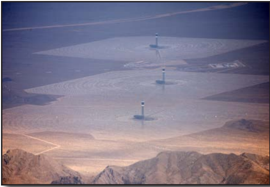
Aerial view Ivanpah Solar Power Facility Photo: Marcus Cyron
